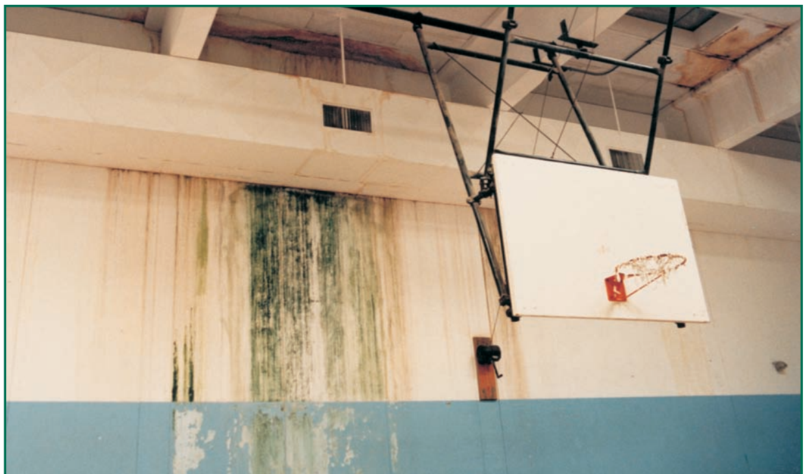
Obvious damage has been done by moisture and mold in this gymnasium.
